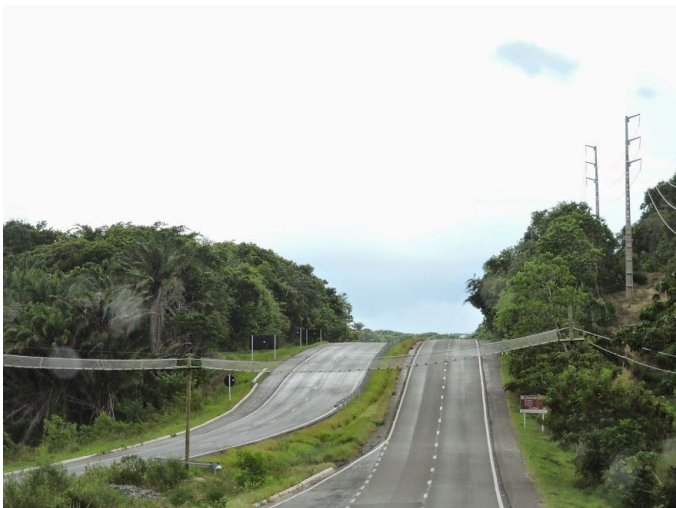
Bridge for monkeys and other animals to cross over the road in Bahia, Brazil
